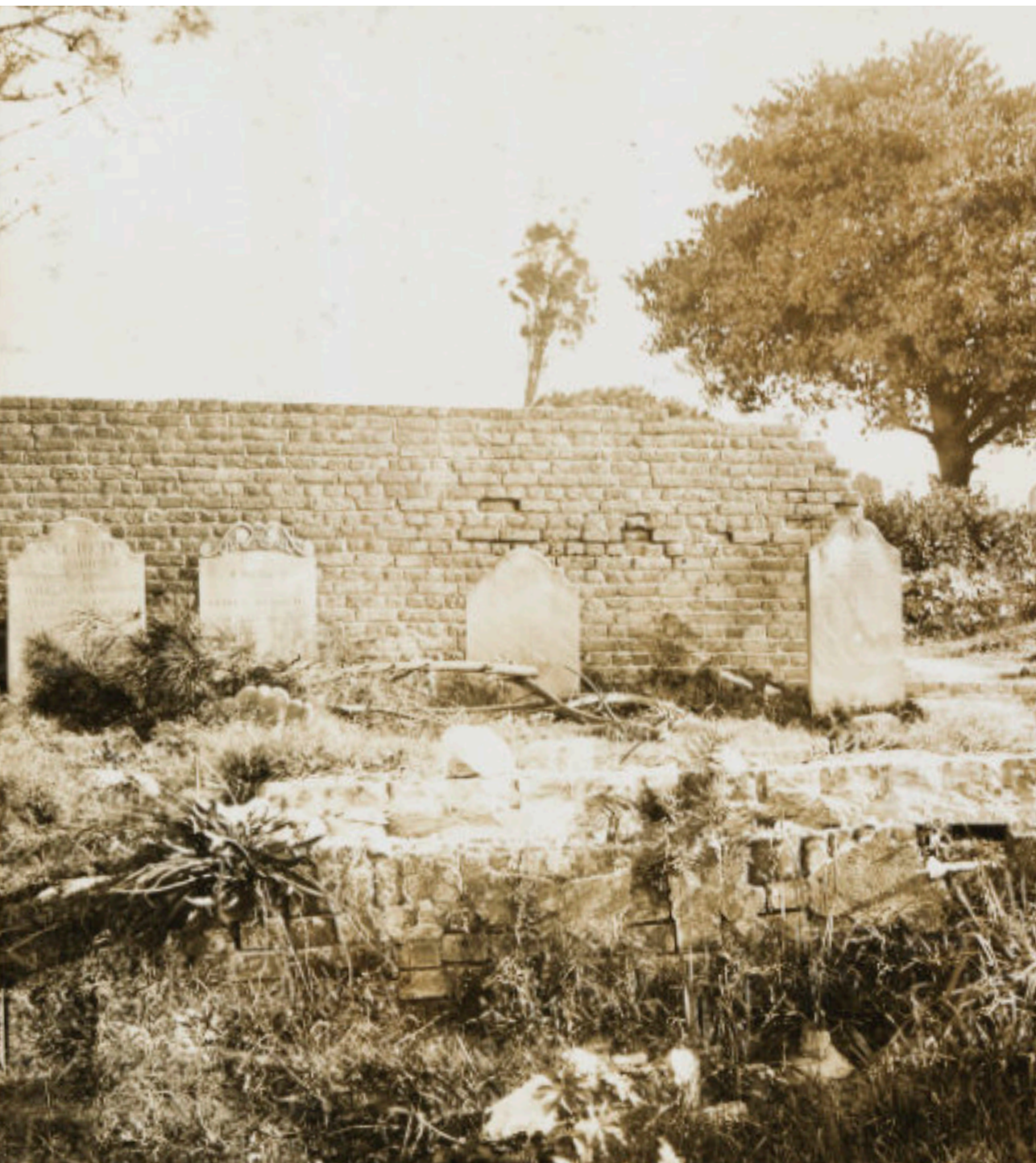
The top half of the headstone can just be made out on the far left of this photo from the c.1900 photograph albums of Mrs Arthur George Foster. SLNSW. Inset: JSR's sketch of the same. SLWA.
